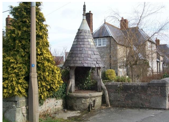
Terfyn Wellhead, Bodelwyddan – a Grade II listed picturesque well of around 1868
