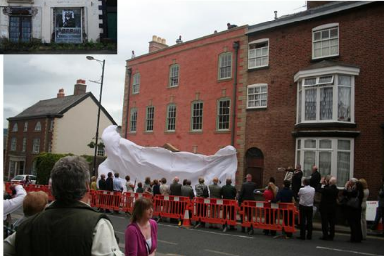
Mostyn House, Vale Street, Denbigh, a Grade II fine town house – historical research and uncovering of features during works returned the character of the building back to its Georgian origins
